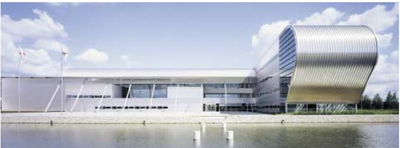
New building of Würth Nederland B.V.; Headquarters of Würth Finance International B.V. in 's-Hertogenbosch NL
